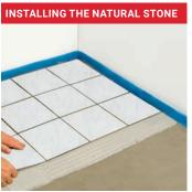
Spread the natural stone adhesive and then lay out and join the natural stone. In wet areas, apply a watertight coating before the natural stone adhesive.
