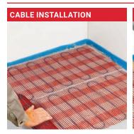
Clean the floor. Apply a layer of adhesive primer. Roll out the heating mat on the floor.
