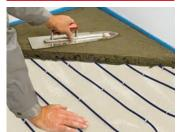
Apply the screed carefully without damaging the heating cable. Let the screed cure according to the manufacturer's instructions.
