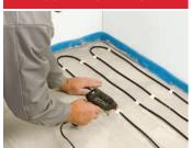
Apply a layer of adhesive primer. Attach the heating cable on the clean floor (e.g. use hotglue gun), or attach the cable directly into anti-fracture membrane.
