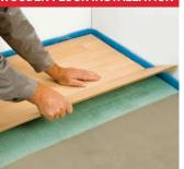
Install the laminate or the wooden floor according to the manufacturer's instructions on the completely cured levelled floor.
