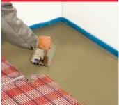
Carefully apply an even layer of filler on top of the mat.
