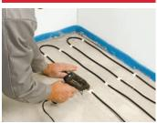
Determine the position of the heating zones before starting the installation of the heating cable and screed layer in agreement with the planner/architect.
