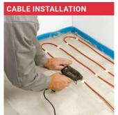
Clean the floor. Apply a layer of adhesive primer. Attach the cable (eg. use glue gun) on the floor.
