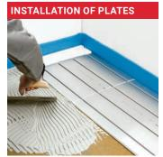
Apply Reflecta Adhesive A-FIX onto the subfloor (or use 15 screws per plate for wooden subfloors). Place the Reflecta plates on top of the glue.
