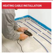
Apply a layer of adhesive primer. Attach the heating cable (e.g. use hotglue gun) on the clean floor.
