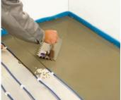
Carefully apply an even layer of levelling compound on top of the heating cable. Let it cure according to the manufacturer's instructions.
