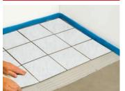
Spread the natural stone adhesive and then lay out and join the natural stone. In wet areas, apply a watertight coating before the natural stone adhesive.
