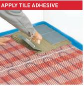
Apply the tile adhesive directly on the QuickNet mat. In wet areas, apply a filler and watertight coating before the tile adhesive.
