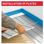
Lay out the Reflecta plates (no need to screw or glue them) on the subfloor.
