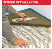
Carefully apply a screed on top of the cable. Let it cure according to the manufacturer's instructions. Depending on the type of screed this process can start after 7 days (anhydrite screed) or 21 days (cement screed). The first heating up and down procedure of the screed has to be agreed with the supplier and documented.
