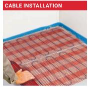
Clean the floor. Apply a layer of adhesive primer. Roll out the heating mat on the floor.
