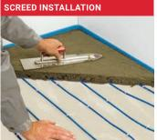
Apply the screed carefully without damaging the heating cable. Let the screed cure according to the manufacturer's instructions.
