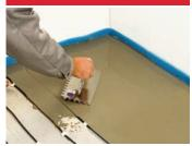
Carefully apply an even layer of levelling compound on top of the heating cable. Let it cure according to the manufacturer's instructions.
