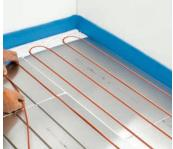
Place the T2Red heating cable in the grooves. The desired heat aluminum layer. output is determined by how closely you space the cable (100, 200 or 300 mm).
