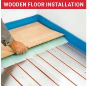
Place a wood floor underlay on top of the Reflecta plates and then lay the new wooden or laminate floor according to the instructions of the manufacturer.
