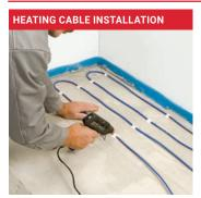
Determine the position of the heating zones before starting the installation of the heating cable and screed layer in agreement with the planner/architect.
