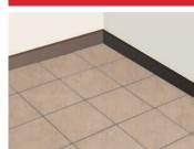
Seal between tiles and walls with a silicon sealant. Allow the floor to cure completely before turning the underfloor heating system on.
