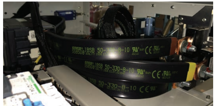
Figure 10 – nVent ERIFLEX IBSB used in tight spaces
