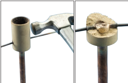
Fig. 16 – Break the ceramic Cadweld One Shot mold off of the connection. Avoid contact with hot materials. See the “nVent ERICO Cadweld Quality Standards” section to see whether a quality connection has been made.
