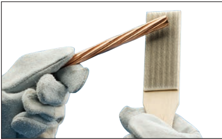
Fig. 12 – Next, use a wire brush to further prepare the surface of the conductors (nVent ERICO T-313 or T-314 brush). Scrape the outer surface to remove dirt and oxidation. You will notice a slight color change.
