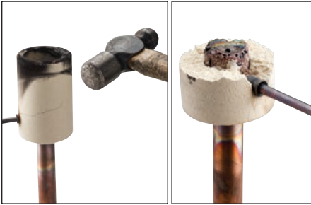
Fig. 15 – Break the ceramic Cadweld One Shot mold off of the connection. Avoid contact with hot materials. See the “nVent ERICO Cadweld Quality Standards” section to see whether a quality connection has been made.
