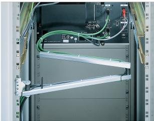
Cable support arm allows pull-out devices and chassis to act as cable management tools. The cables would be bundled together using cable ties.
