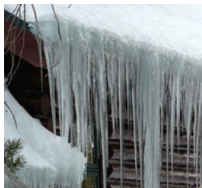
Unprotected roof and gutters
