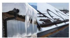
High quality and quick-to-install cable systems for keeping gutters and downspouts free from snow and ice. This heating solution prevents icicle formation and damage to gutters and ensures water can keep flowing freely.
