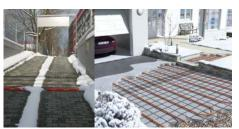
Effective and reliable heating systems for keeping driveways, stairs and footpaths free from snow and ice. This heating solution prevents physical injury and vehicle accidents, and saves time clearing snow.
