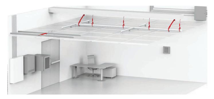
To help ensure the availability and operation of safety systems after an earthquake event, many building and industry codes now include requirements for the design and installation of seismic sway bracing for non-structural components, such as fire sprinkler, mechanical, electrical and plumbing systems.
