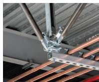
Trapeze Sway Brace, Pipe, CSBR1
