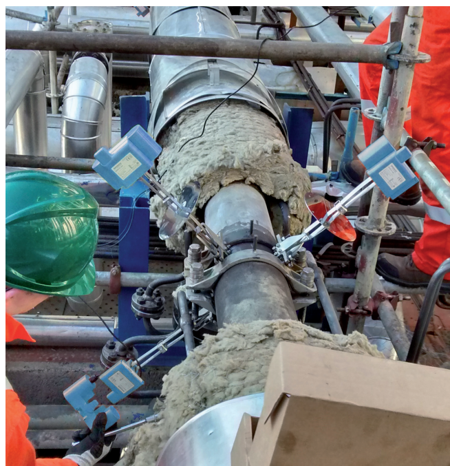
Figure 6 Example installation of Rosemount WT210 Transmitters
