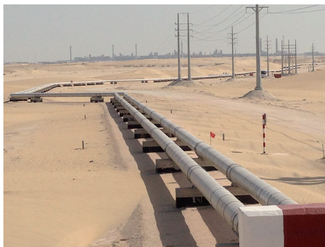
Figure 2 Raychem longline heating system
