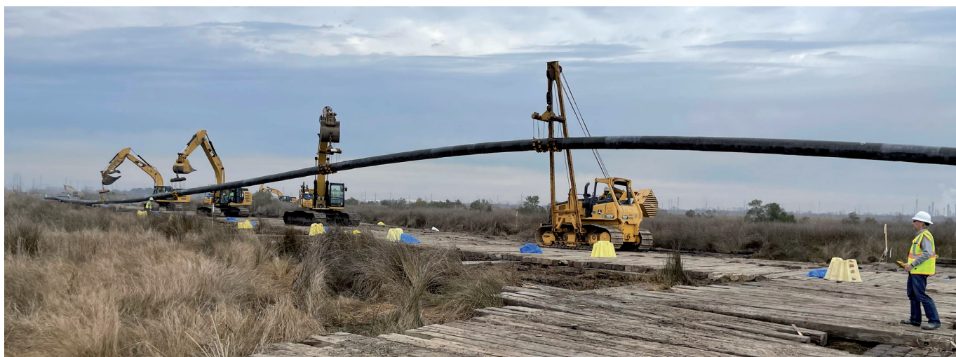
Figure 5 STS longline heated pipeline
