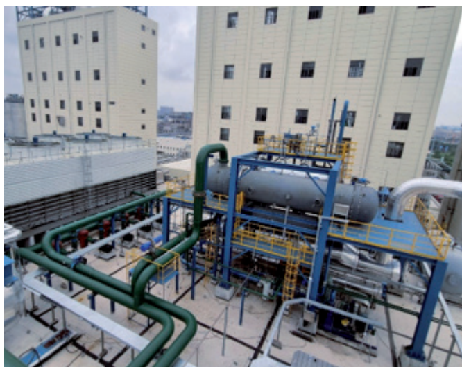
Figure 5 Overview of Exergy's ORC waste heat recovery installation at Sanfame's chemical plant
