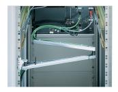
Cable suport arm allows pull-out devices and chassis to act as cable management tools. The cables would be bundles together using cable ties.
